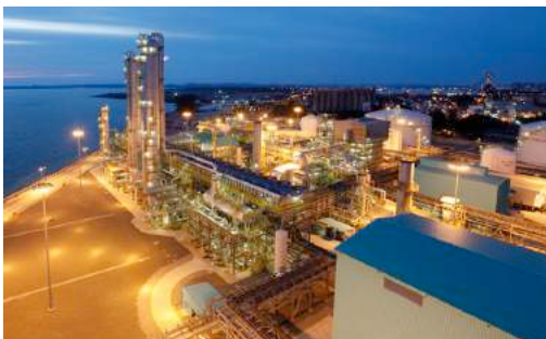
Ethylene Oxide and Ethylene Glycol (MEOG) Plant, Kertih, Kuala Terengganu
