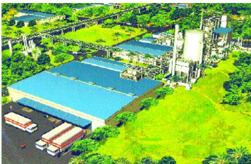
PVC Paste Plant construction and extension for Kaneka Sdn Bhd, Gebeng
