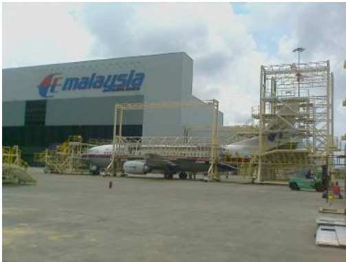
Docking system in Hangar 6 for Malaysian Airline Systems (MAS), Kuala Lumpur International Airport
